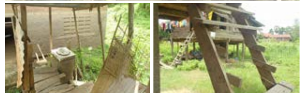
Many survivors are living under the conditions with no walls or floorboards, broken latrines and inclined pillars
