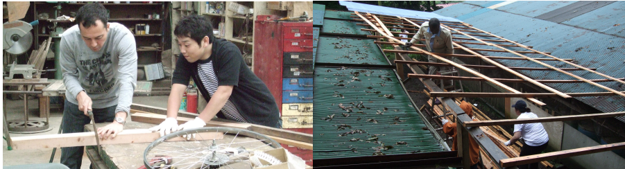
Left above) Working on the Bench, Right above) Working on the Poultry House roof
